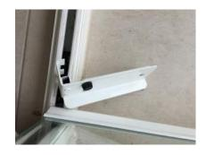
Push the wedge, hooks down, into the track, until flat. in line with the glass door edge.
